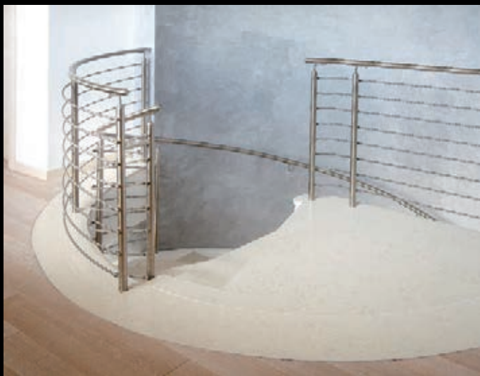
Concrete helical staircase (diameter 260 cm)
