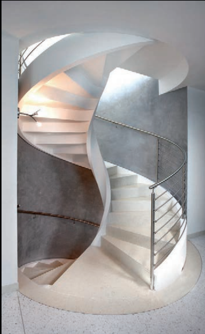
Scala elicoidale in cemento (diametro 260 cm)
